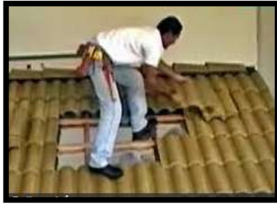
THERE 'S A MAN ON THE ROOF.
